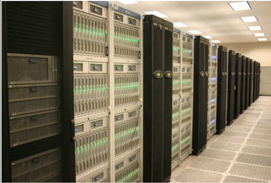
Figure 1. One of 6 rows: Management/IO Racks (black), Compute Rack (silver), and In-row Cooler (black).
