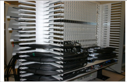
Figure 3. Constellation Switch (partially wired).
